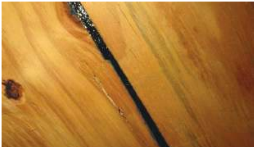
SWR installed under the metal panels
